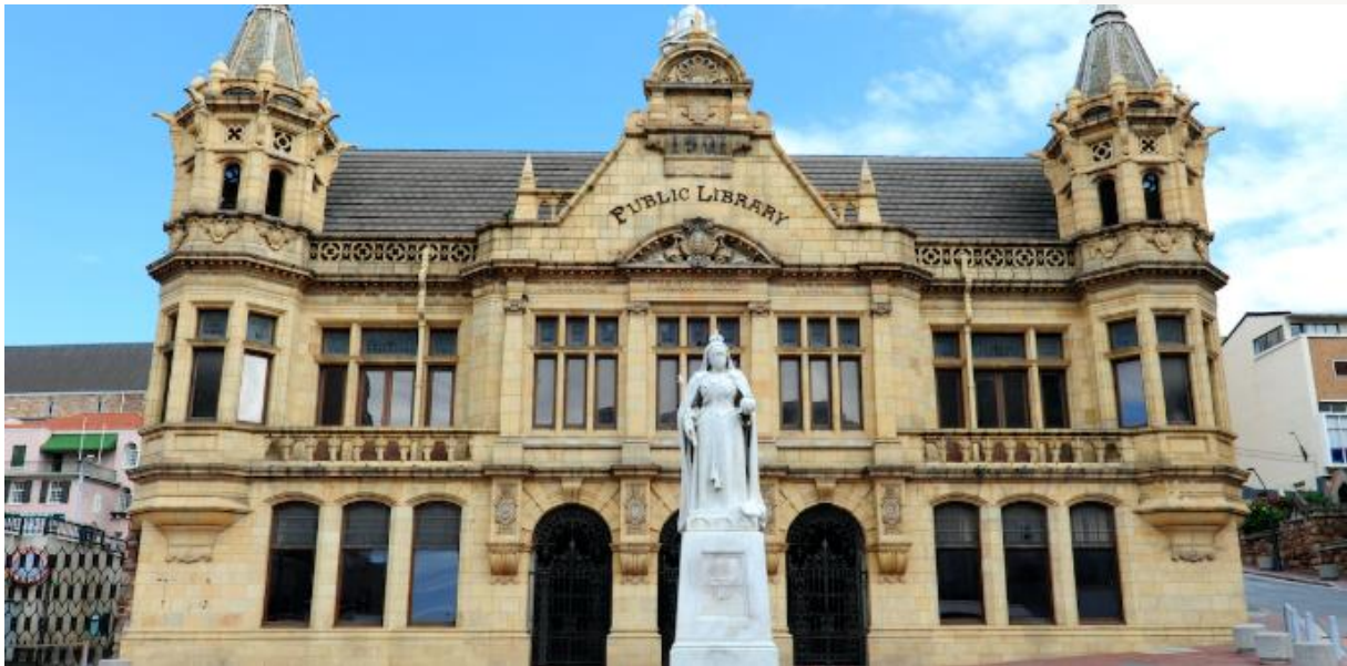
The Port Elizabeth Library: A National Monument
